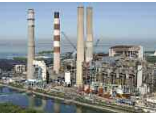
Above: Tampa Electric's Big Bend Power Station .
